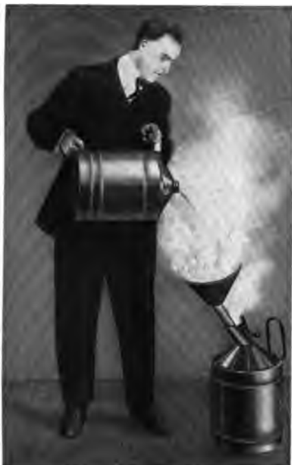
Fig. 1. Man Pouring burning Gasolene from one Safety Can to another.
